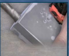
Counter-Sink Holes: Drill a counter sink hole at the injection port to accept injector tip approx 1/2" deep.
